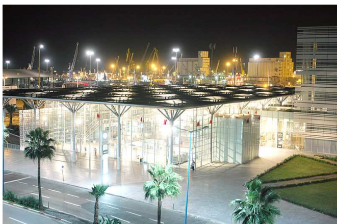
Casa-Port train station (Source: © RogerCageot - Commons.Wikimedia.org)
